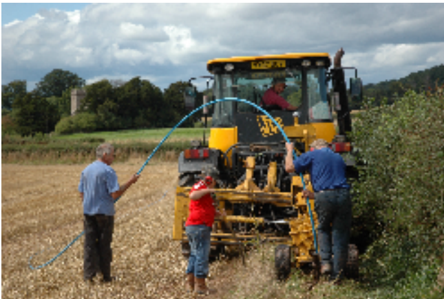
The photograph shows the pipe being laid.
